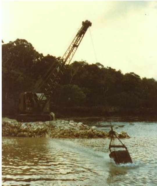
Excavator Track Mounted 22 RB Rigged as a dragline Cikobia FIJI 1983 Jack Madden photo
